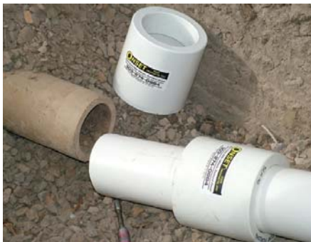
Step 1 Slide the Shear Guard® support onto 4" exposed plastic pipe that is to be joined to existing clay pipe.
