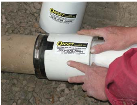
Step 3 Slide the Shear Guard® support into place over flexible coupling aligning clamp screw into key hole.
