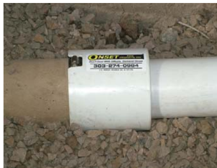
Step 4 A Properly installed Shear Guard® support; bedding and backfill per local codes.
