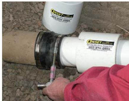
Step 2 Attach flexible coupling to pipes then tighten both bands.
